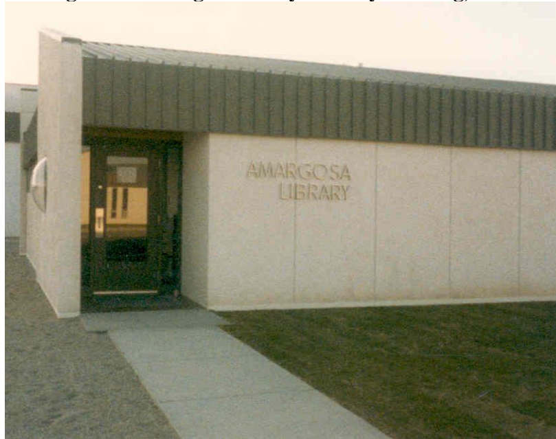
Figure 3: Amargosa Valley Library building, 1984
