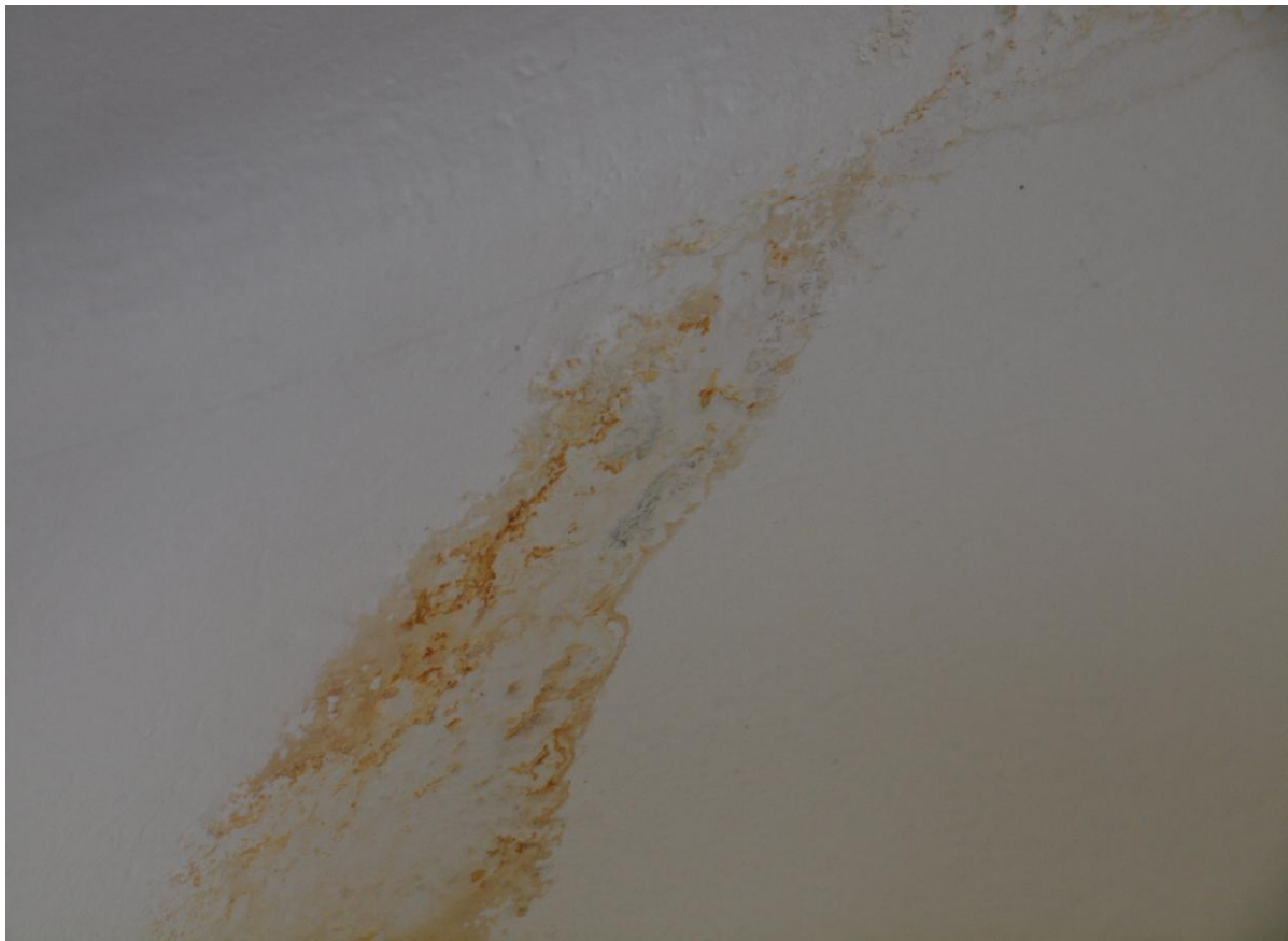
Figure 2. After few days greenish shades appeared. It is an evidence of mould growth, probably of
