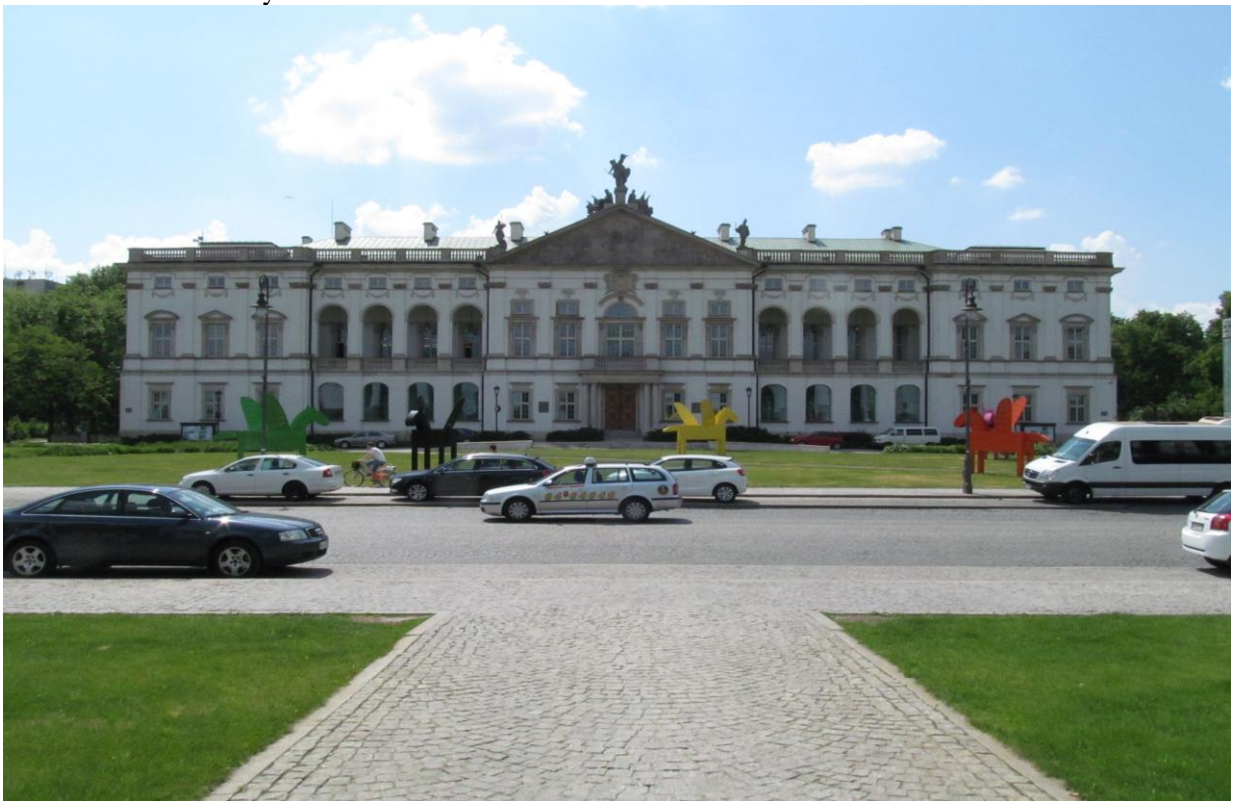
Figure 5. View of the Palace from the Krasinski Square. The two right windows above the second level of arcades just left to the tympanum are the windows of the storage room 218. The water activity appeared on the wall that separates room 218 from the Wilanowska Hall (five
