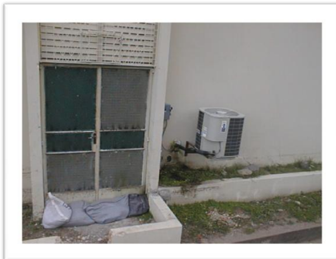
Fig.12 Using sandbags in a flood prone area
