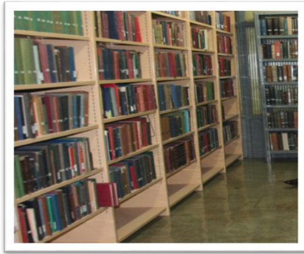
Fig.9 Discontinuation of shelving on the bottom shelf
