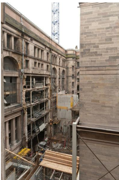
Fig. 5: Work going on in the inner courtyards (oct. 2011)
