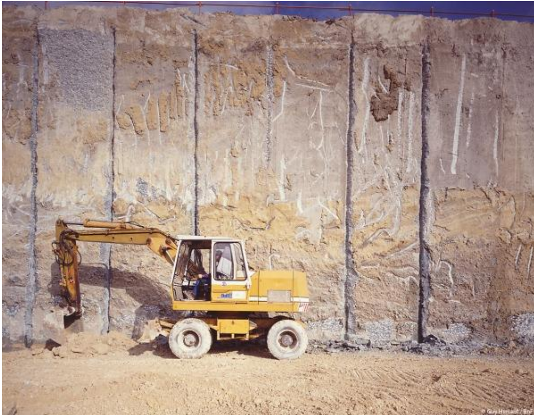
2 Details of the concrete wall
