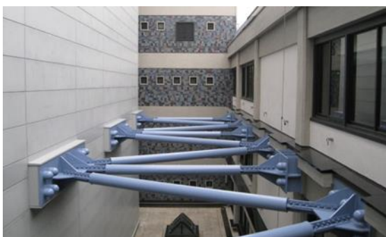
(Fig. 9) Steel braces connecting the stacks and the office building
