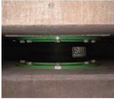
(Fig. 3) Laminated rubber isolator
