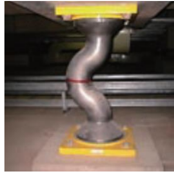
(Fig. 4) Lead damper
