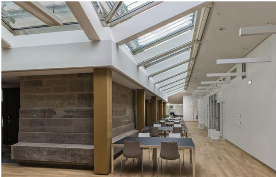
Pic. 3: View of the level 6 reading room. To be seen: preserved historical walls, anti-seismic pillars.
