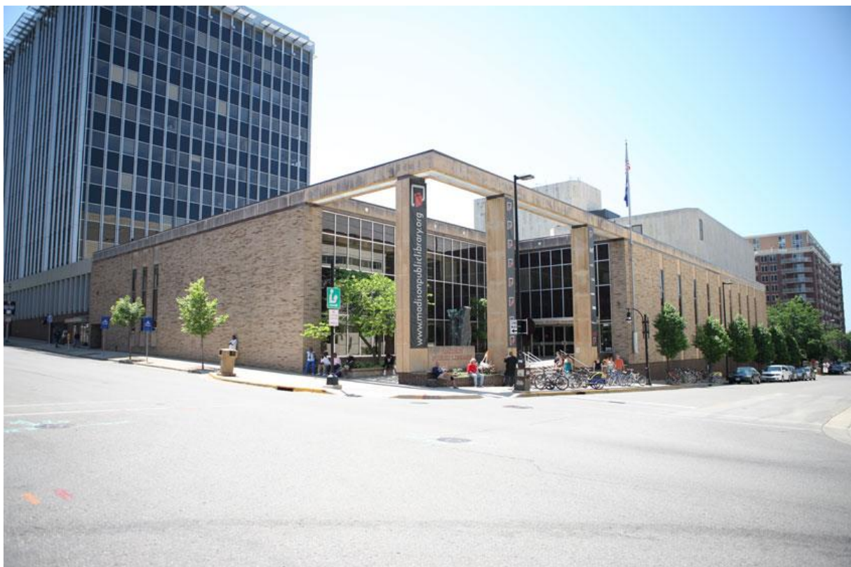
Figure 1: The existing building was often referred to as a “ de facto homeless shelter” (Photo: MSR).
