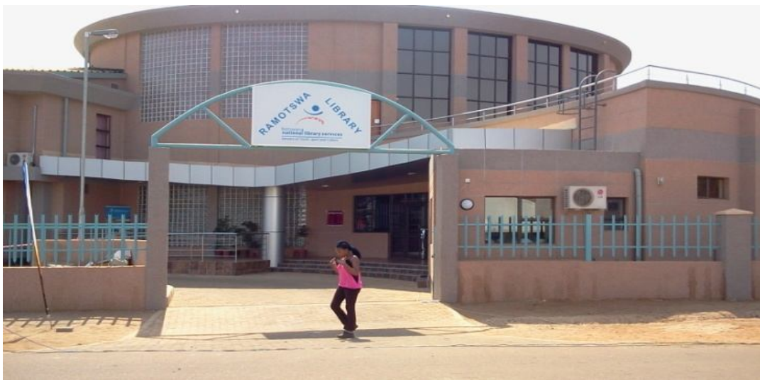
Ramotswa Public Library – one of the new library buildings
